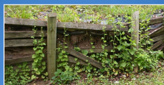
House with sagging foundation and cracked walls
